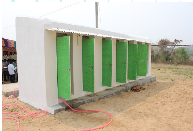
Outdoor bathroom and shower facilities of the Siloam Home
